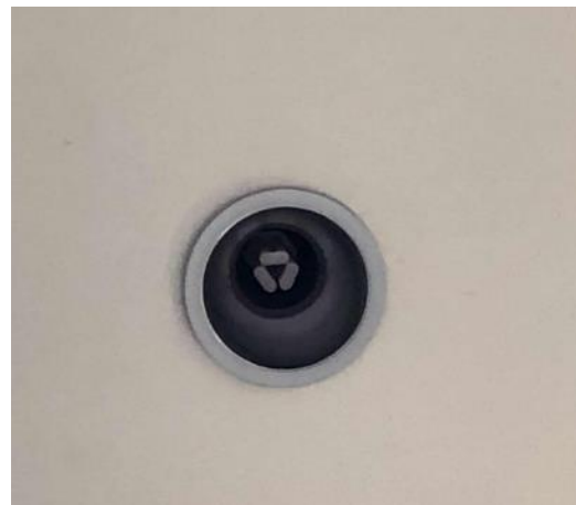
Recessed Can Fixture
