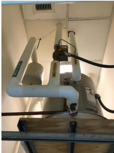
DHW Storage Tank Water Heater
