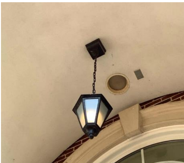
Pendant Mounted Fixture
