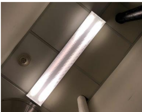
Surface Mounted Fixture
