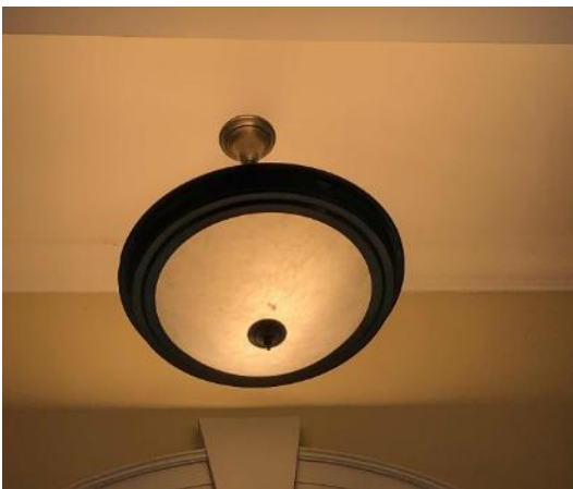
Pendant Mounted Fixture
