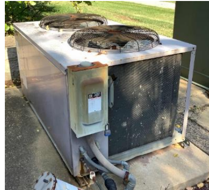
Split System Condensing Unit
