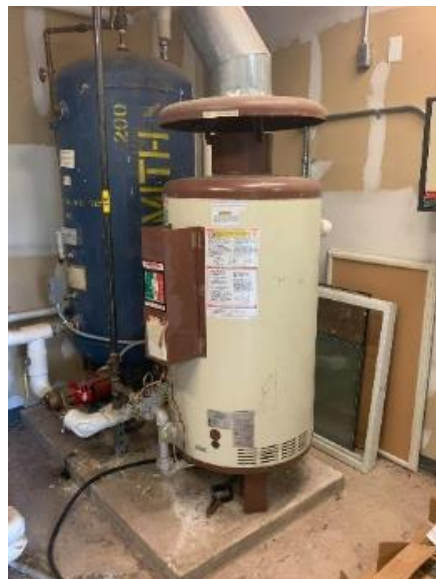
Gas Fired Boiler
