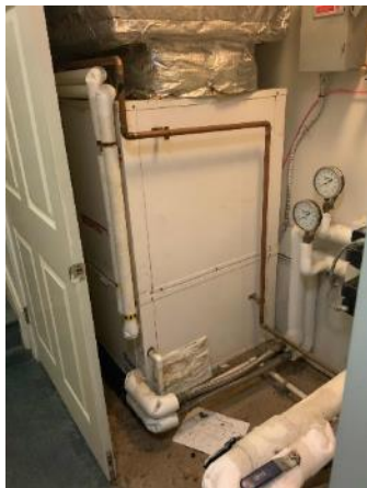
Water Source Heat Pump
