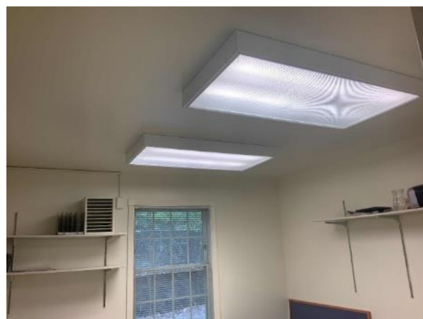
Linear Fluorescent T8 Fixture
