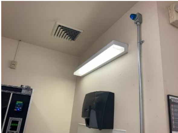
Linear Fluorescent T8 Fixture
