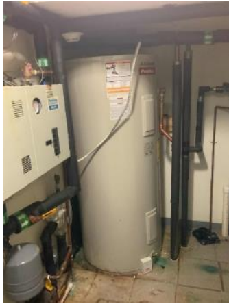
Electric DHW Tank
