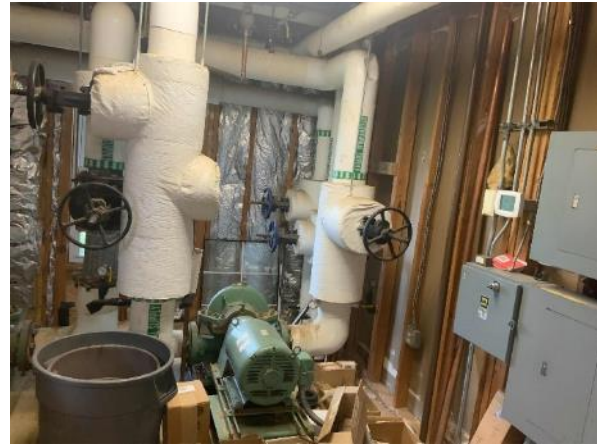
Geothermal Pump
