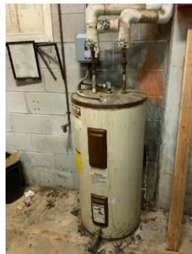
Electric DHW Storage Tank
