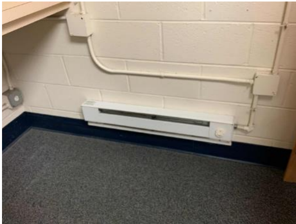
Electric Resistance Heater
