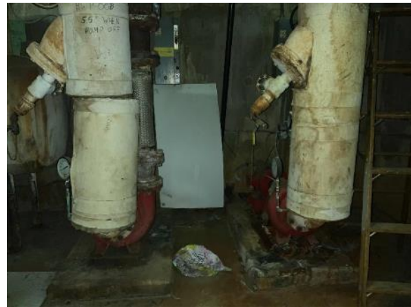
Heating Hot Water Pumps
