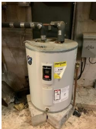
Electric DHW Storage Tank
