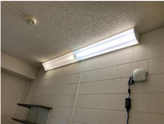
T8 Linear Fluorescent Fixtures
