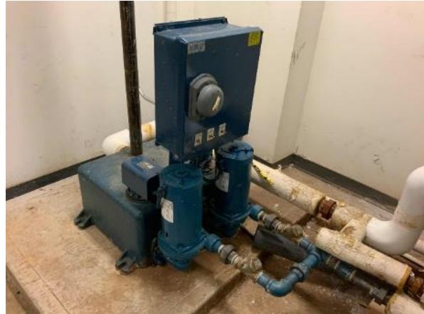
Steam Condensate Return Pumps
