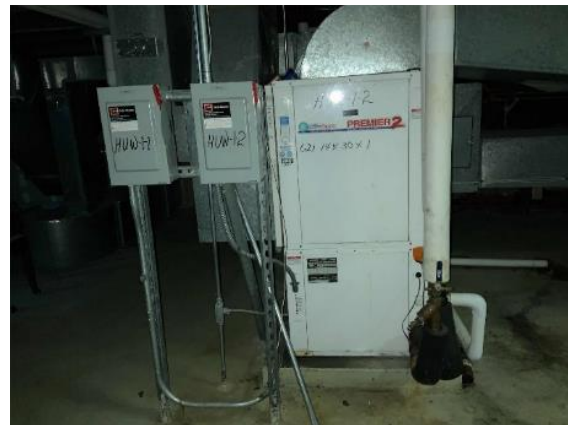
Waterfurnace Heat Pump
