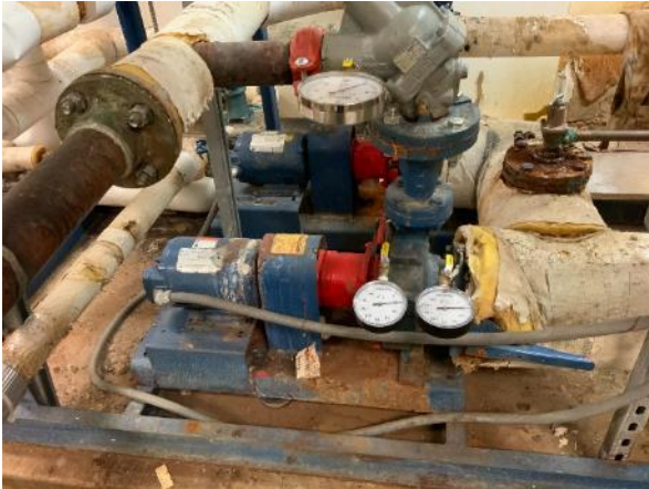
Heating Hot Water Pumps
