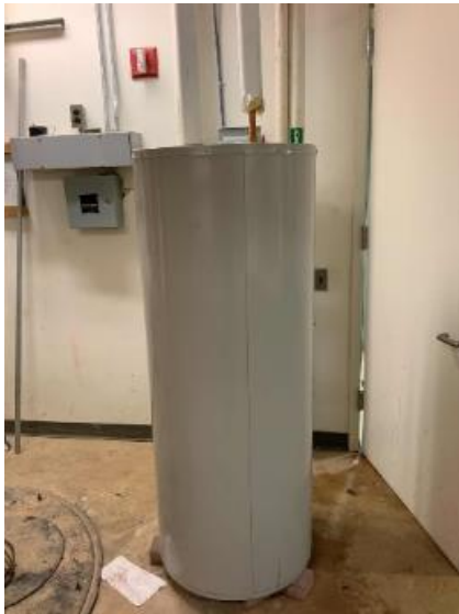
Electric DHW Tank
