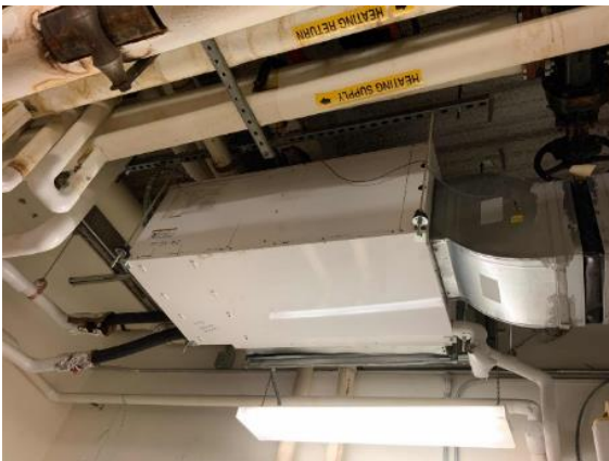
Waterfurnace Heat Pump
