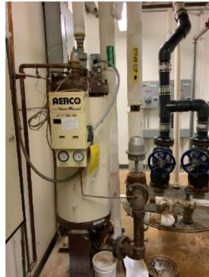
Semi-Instantaneous DHW Heater
