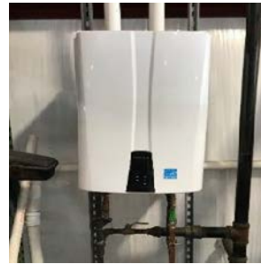
New Building DHW Heater
