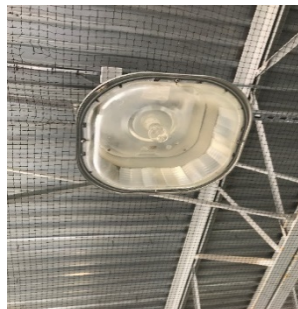
Garage Metal Halide Fixture
