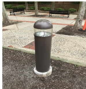
Bollard LED Fixture
