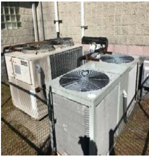
20-ton and 15-ton split AC units
