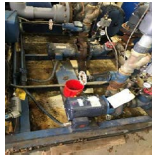
Heating Hot Water Pumps
