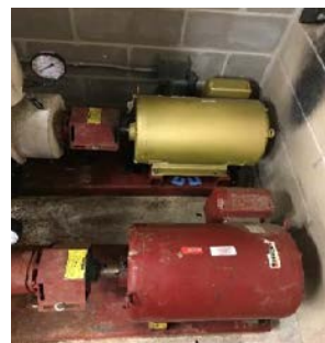
Condensing Water Pumps
