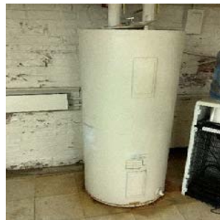
Electric domestic hot water heater
