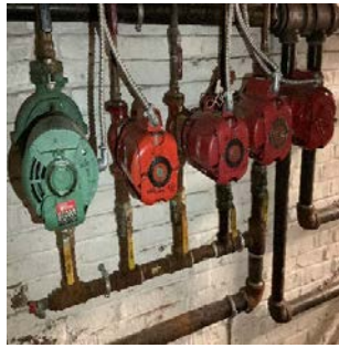
Hot water circulation pumps
