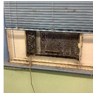
Window AC in poor condition
