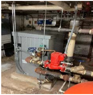
Condensing type hot water boiler
