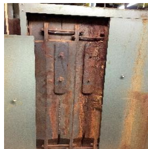
Boiler internal parts rusted
