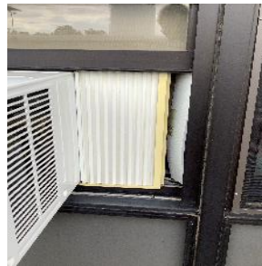
Window AC with poor insulation
