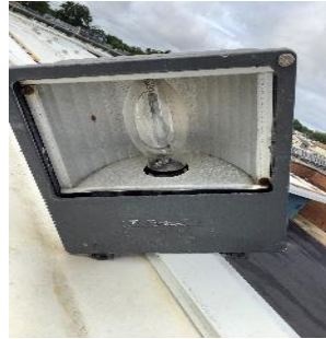
Wall-mounted fixture with metal halide lamp
