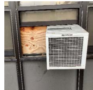
Window AC with wooden plank as insulation
