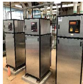
RBI condensing type boilers
