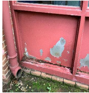
Panel below windows in poor condition
