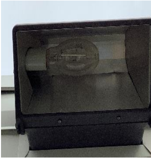
Wall-mounted fixture with metal halide lamp
