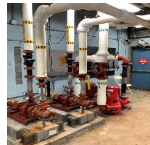
Heating hot water pumps
