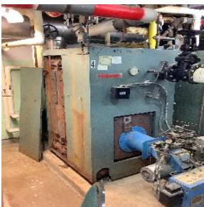
HB Smith cast iron boiler
