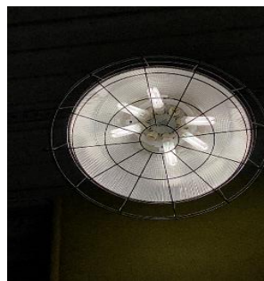
6-lamp fixture in Gym with CFLs
