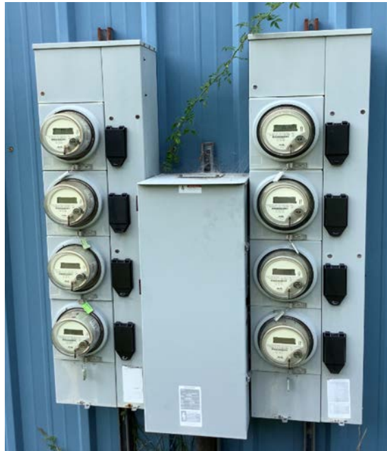
A-Hangar Associated Electric Meters (Mix of Borough & Other Utility Accounts)
