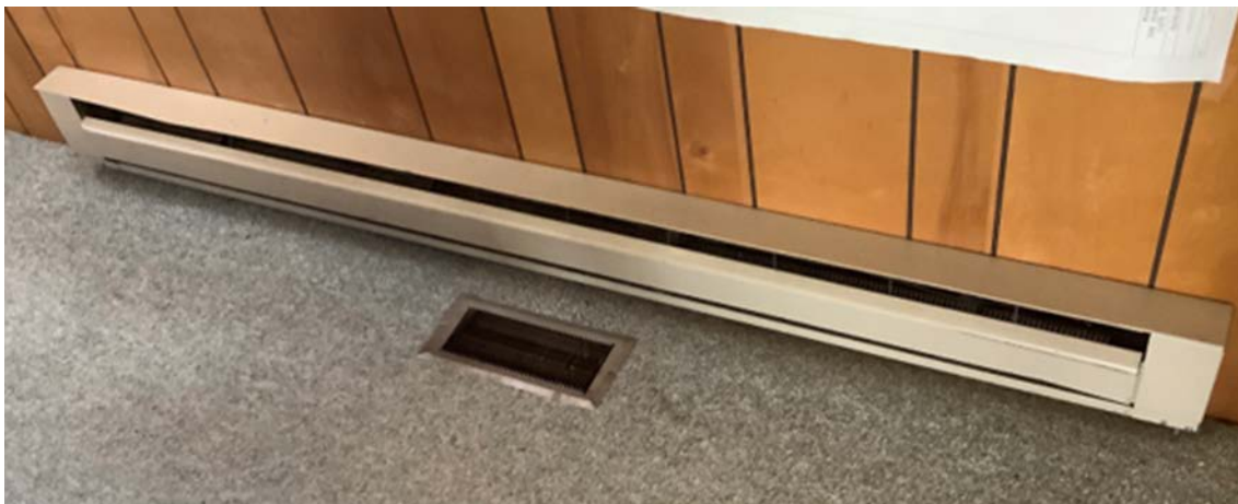
Electric Resistance Baseboard Heater
