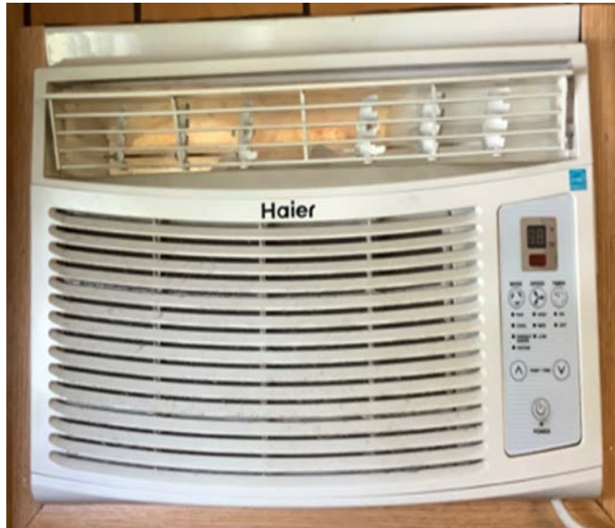
Programmable Thermostat & Haier Window Unit
