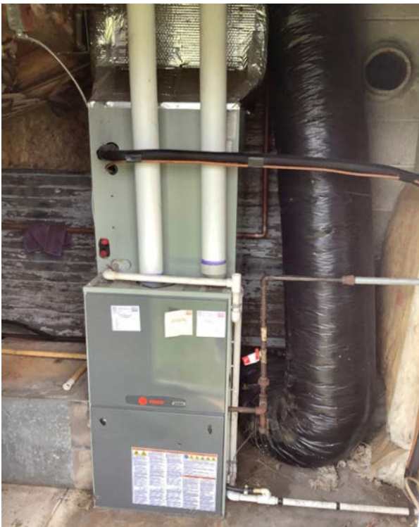
Trane Furnace & Condensing Unit
