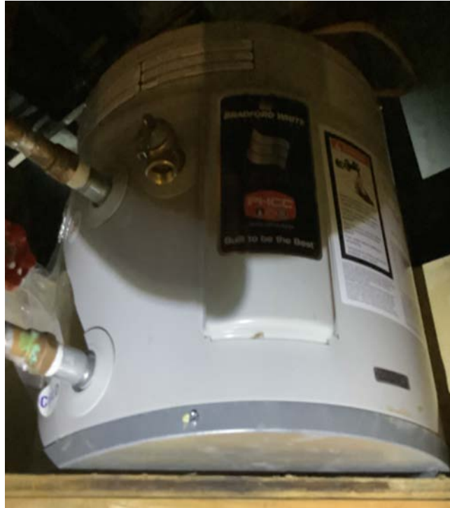
Electric Storage Tank Water Heater
