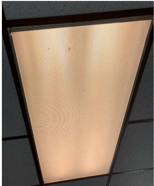
Linear Fluorescent T8 Fixtures
