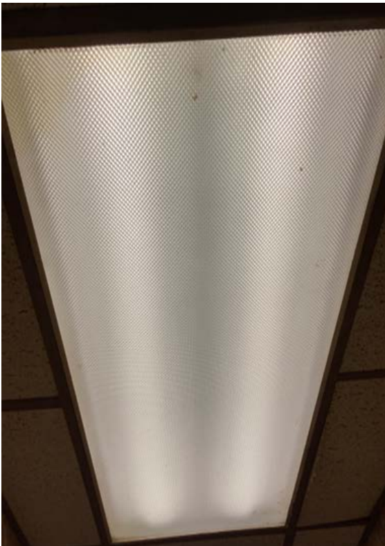
Linear Fluorescent T8 Fixtures
