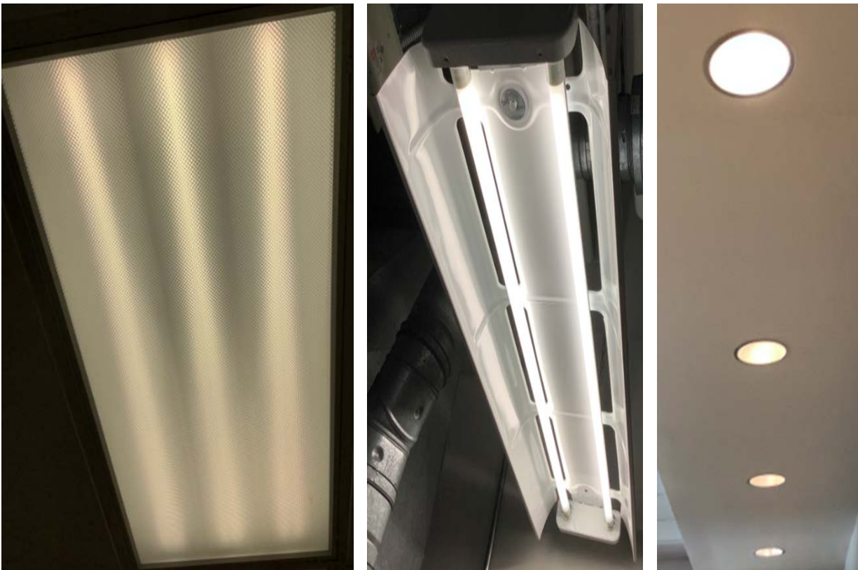
4-Foot Long LED Tubes & LED Screw-In Lamps
