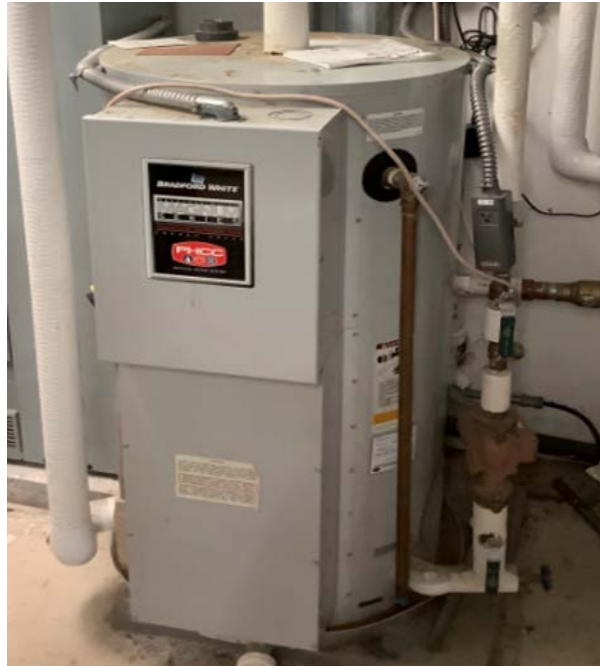
12 kW Electric Storage Tank Water Heater
