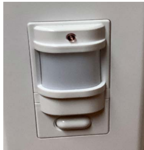
LED Exit Sign & Wall Mounted Occupancy Sensor
