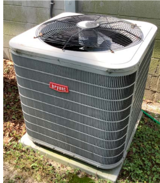
Carrier & Bryant Exterior Condensing Units
