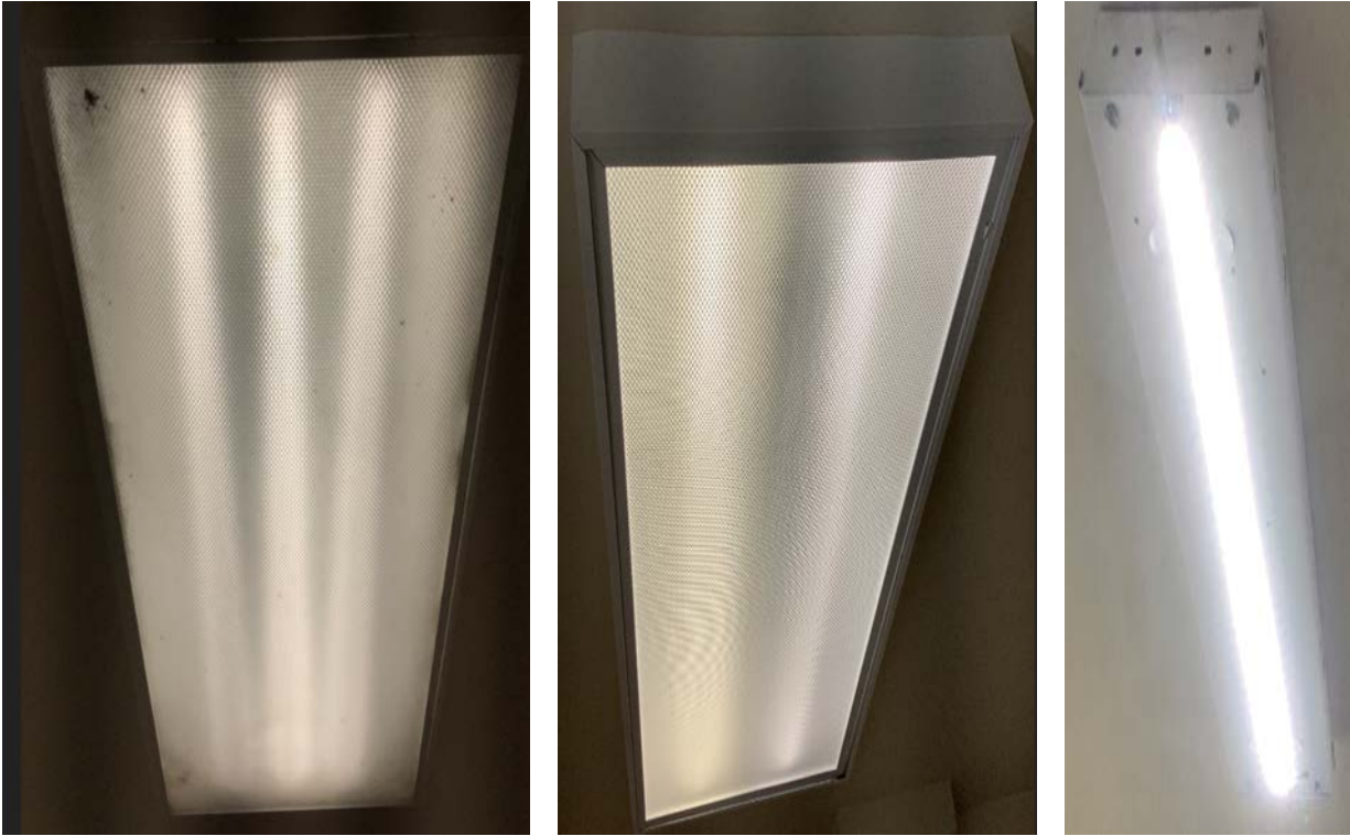
Linear LED Tubes & Strip Fixtures
