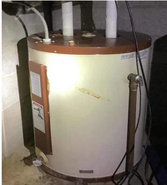
30 -Gallon Storage Tank Electric Water Heater
