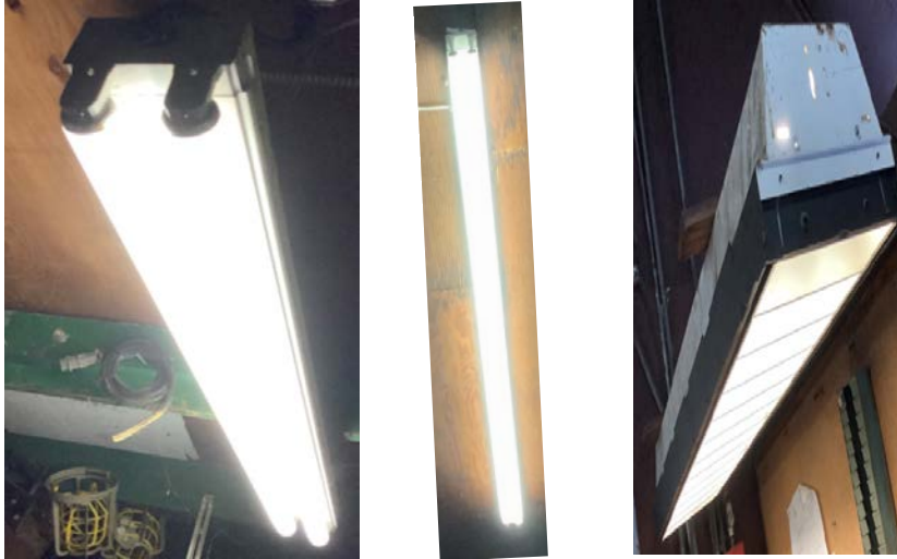
Linear Fluorescent T12 & T8 Fixtures
