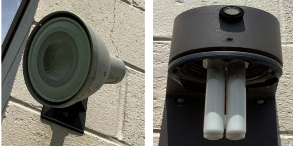
LED & CFL Exterior Fixtures
