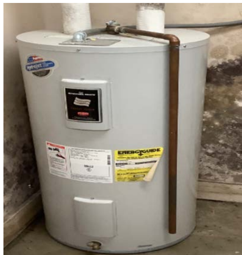
Electric Storage Tank Water Heater
