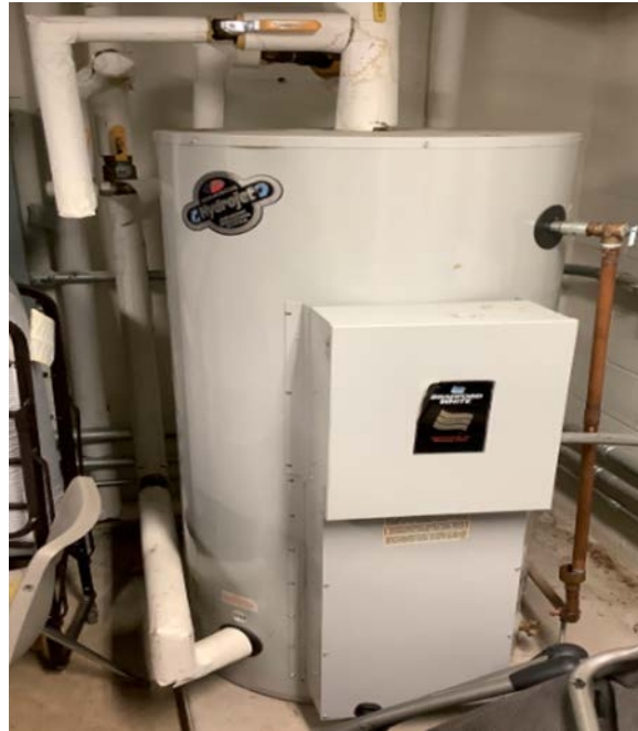
Electric Storage Tank Water Heater
