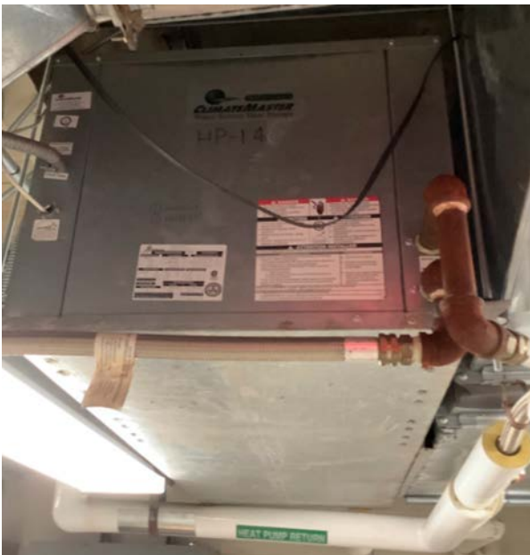
Water Source Heat Pump
