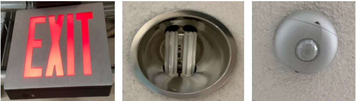
LED Exit Sign, Compact Fluorescent lamps & Occupancy Sensor
