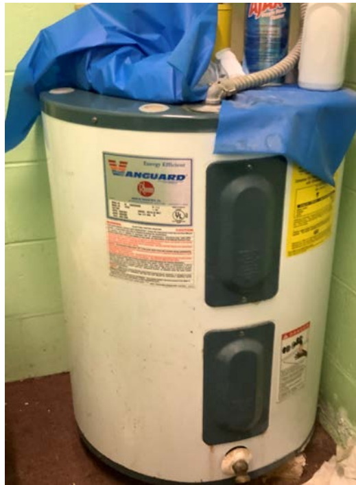
Electric Storage Tank Water Heater
