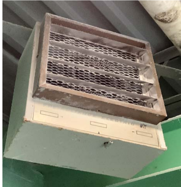
Electric Resistance Heaters
