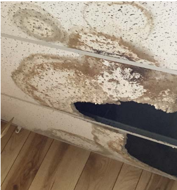
Signs of Ceiling Damage (Roof Leaks) - Office Building
