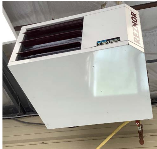
Gas-Fired Warm Air Unit Heaters
