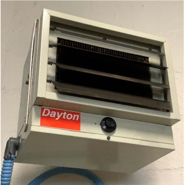
Electric Resistance Heaters
