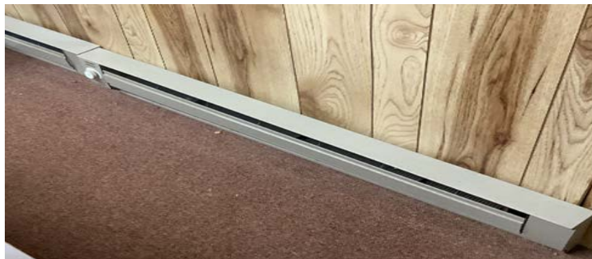
8-Foot Electric Resistance Baseboard Heat
