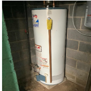
Gas-fired Domestic Hot Water Storage Tank
