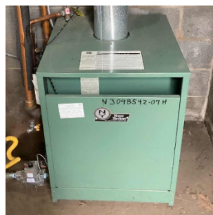
Gas-fired Hot Water Boiler
