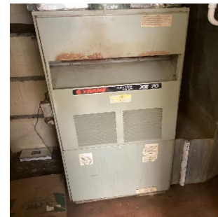
Gas-fired Furnace
