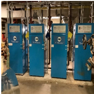
Hot Water Boiler
