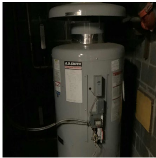
Domestic Hot Water (DHW) Boiler, Unit Label
