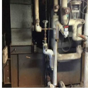
Air Handling Units (AHU)
