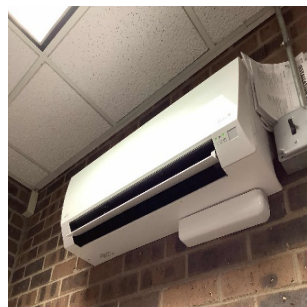
Split Air-Source Heat Pump (HP)
