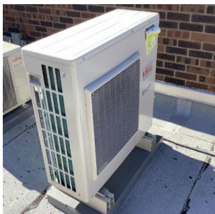
Split Air-Source Heat Pump (HP)
