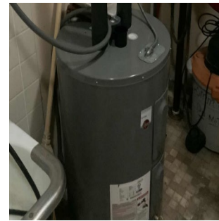
DHW Storage Tank Heater
