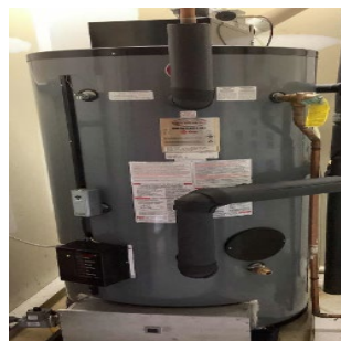
Gas-fired Hot Water Storage
