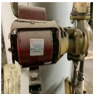
Domestic Hot Water Circulation Pump
