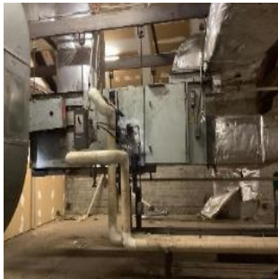
Air Handling Units Located in Mechanical Rooms
