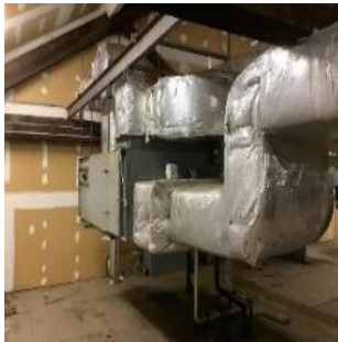
Air Handling Units Located in Mechanical Rooms
