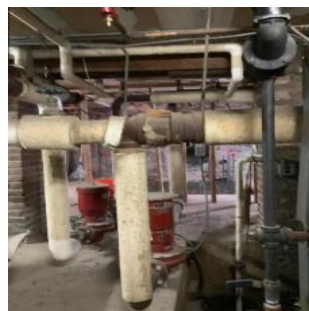
Hot Water Circulation Pumps
