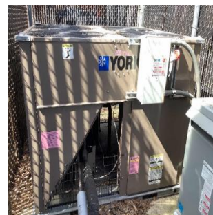
Split system condensing units
