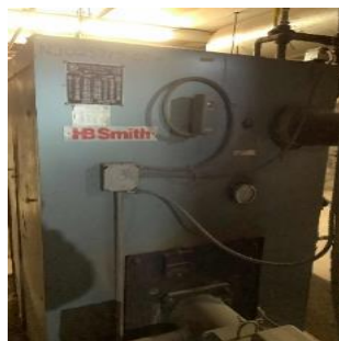
Hot Water Boiler
