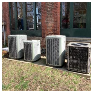
Split system condensing units
