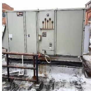
Gas-fired packaged RTU
