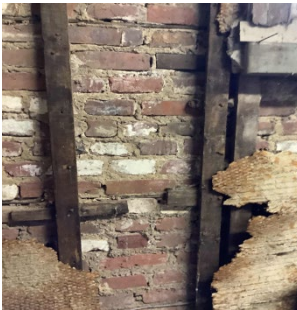
Signs of Interior Wall Damage
