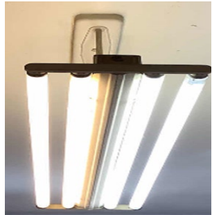
4-Foot Long Linear T12 Fixtures
