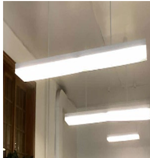
8-Foot Long Linear T-12 Fixture
