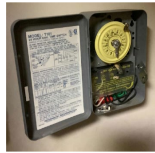
Exterior Timer Lighting Controls
