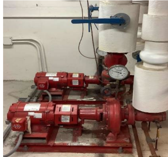
Hot Water Boiler & Heating Hot Water Pumps
