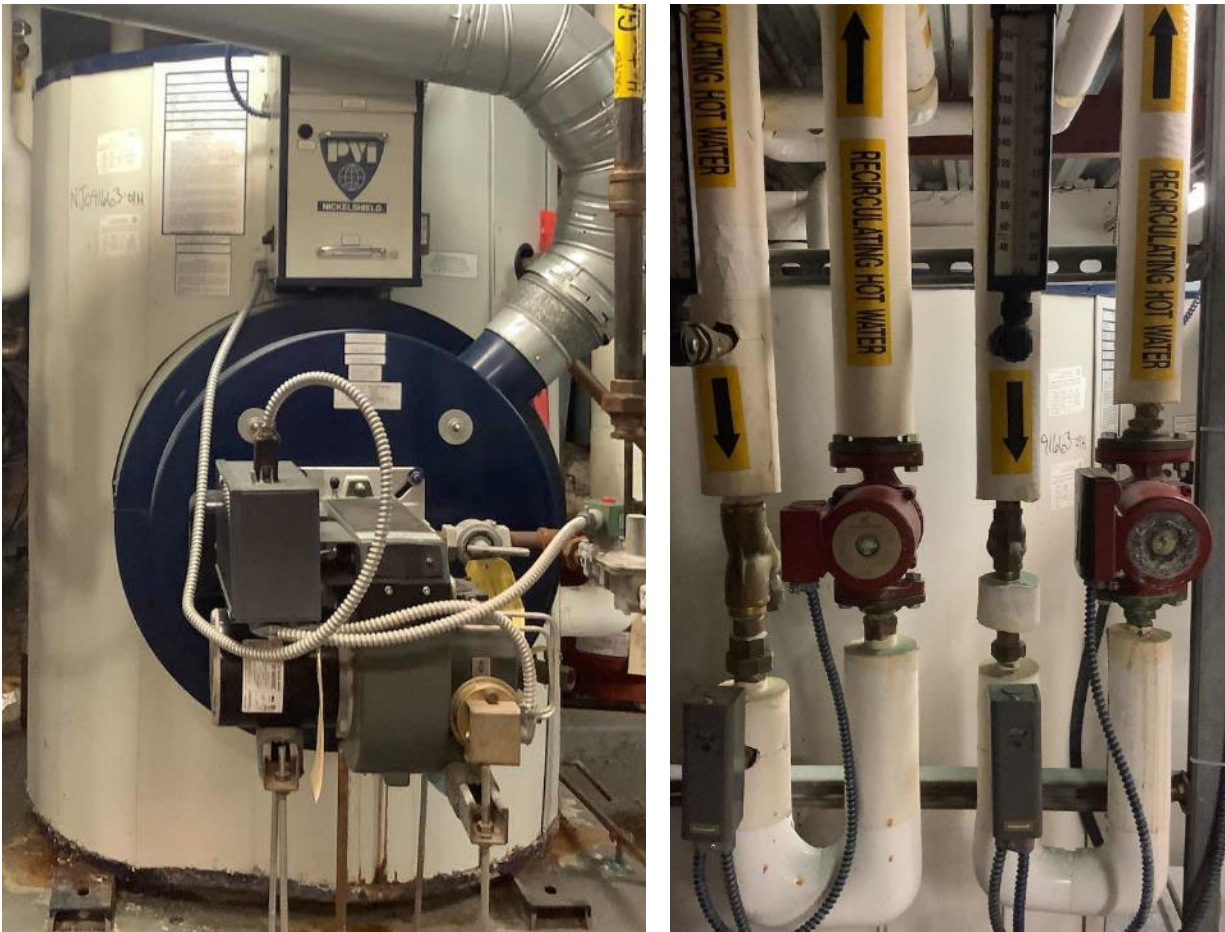
Gas-fired Storage Tank Water Heater & Circulation Pumps
