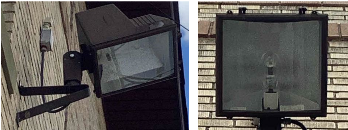
Exterior HPS Fixtures
