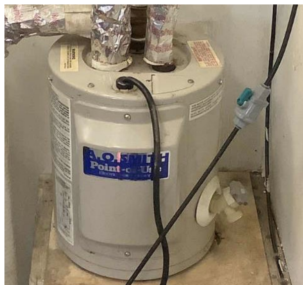
Electric Storage Water Heaters
