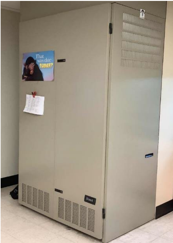
Unit Ventilator & Controls
