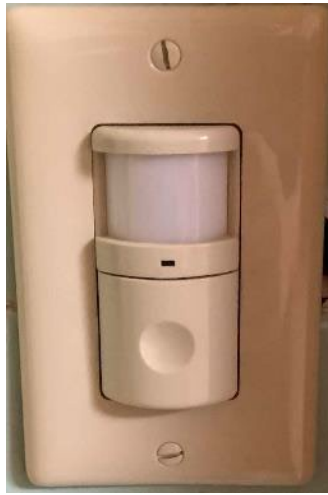
CFL Lamps & Occupancy Sensors
