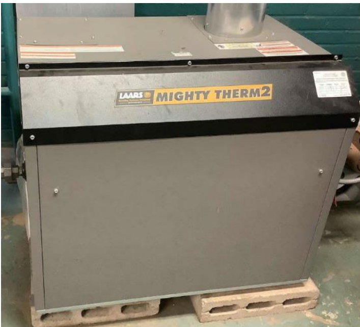
Gas-fired Boiler & Circulation Pump
