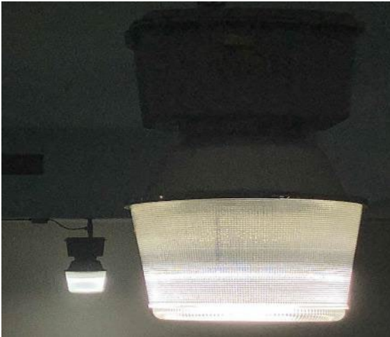
Natatorium High Bay and Wall Pack LED Fixtures
