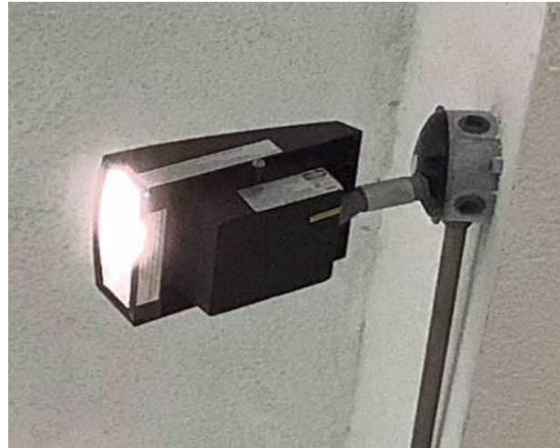
Natatorium High Bay and Wall Pack LED Fixtures
