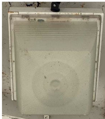
Exterior MH & CFL Fixtures
