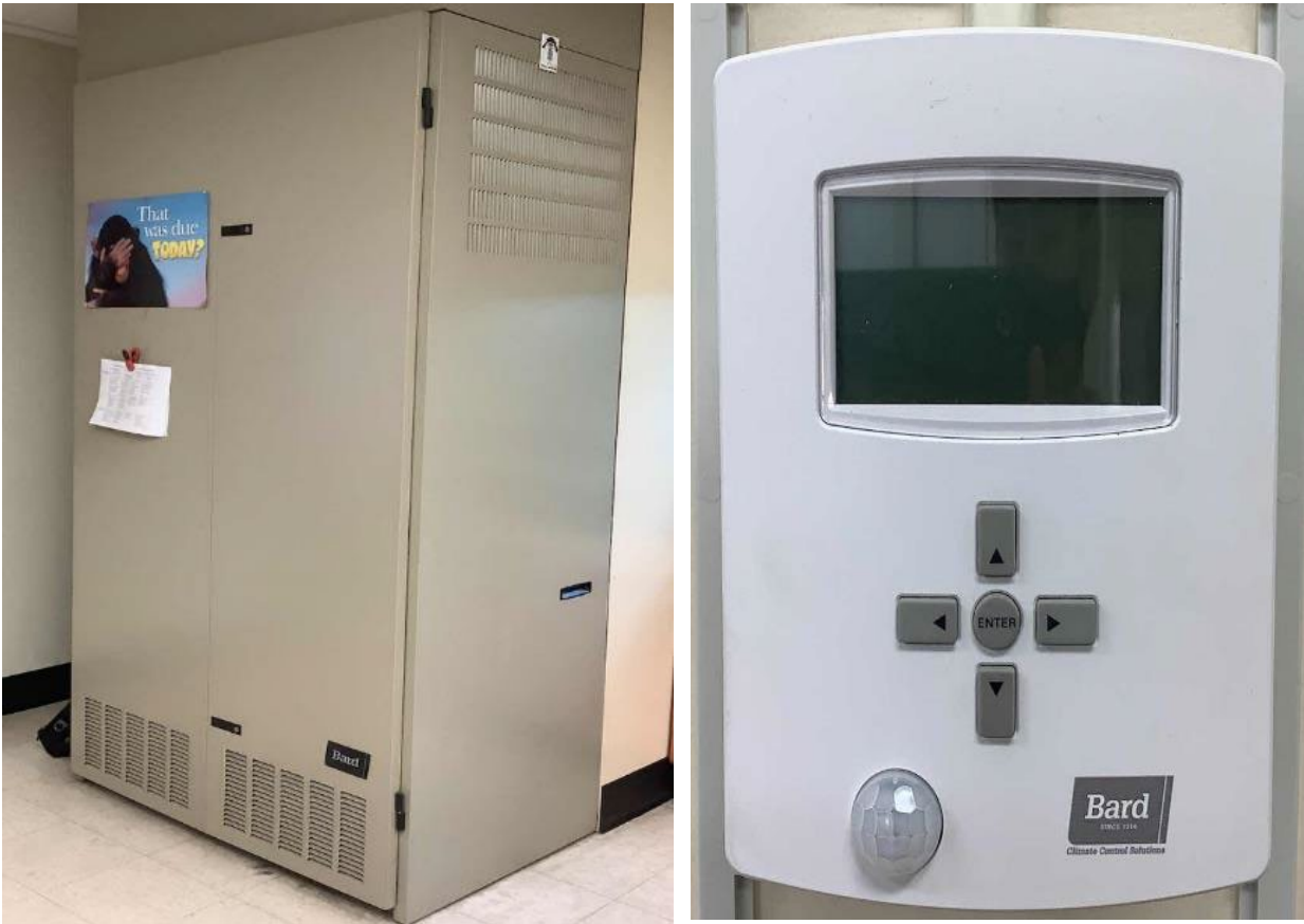
Unit Ventilator & Controls
