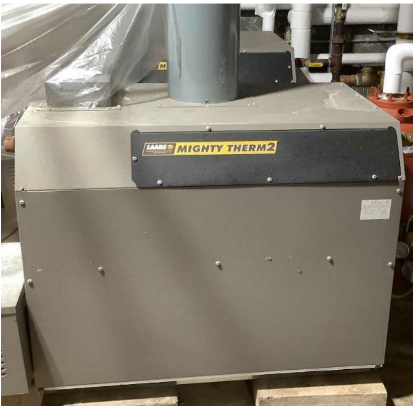
Gas-fired Boiler & Circulation Pump
