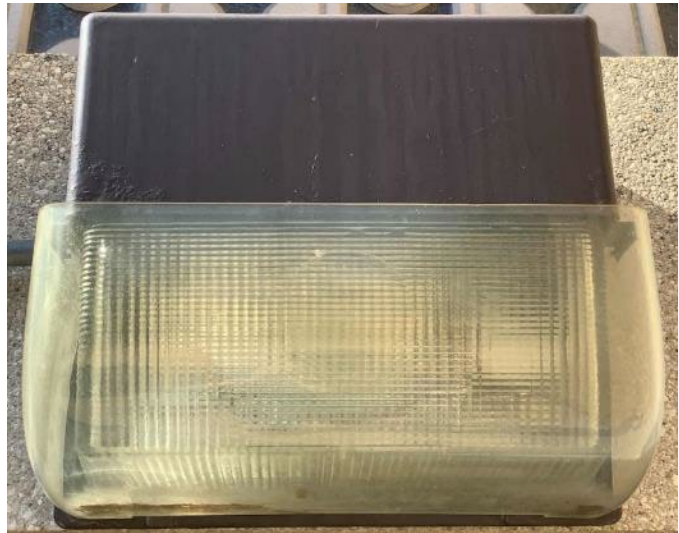
Exterior CFL & HPS Fixtures
