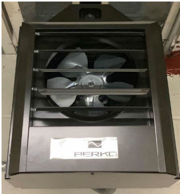
Electric Resistance Heaters
