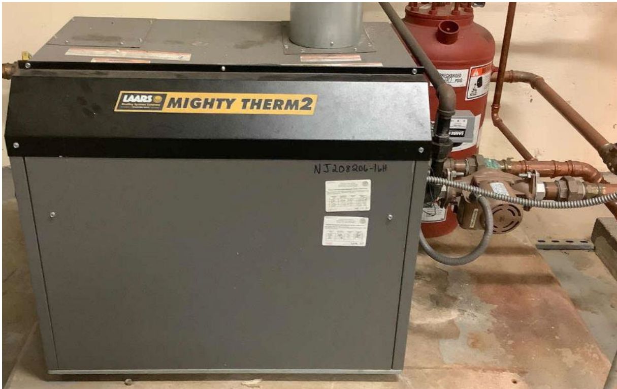
Gas-fired Boiler & Circulation Pump
