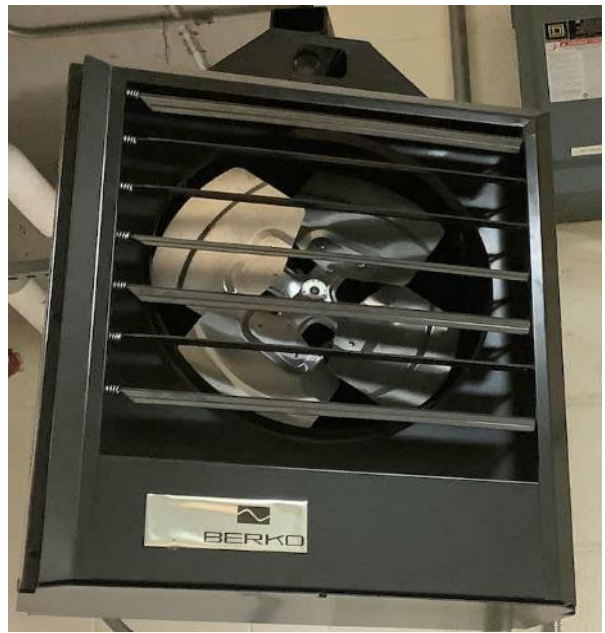
Electric Resistance Heaters
