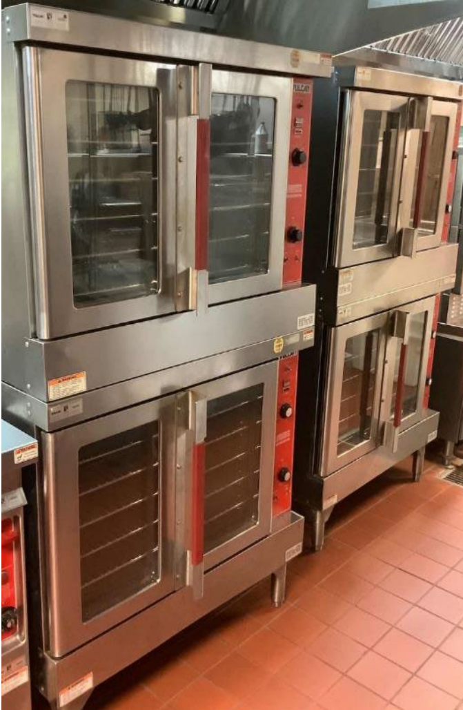
Gas-fired Convection Ovens & Electric Holding Cabinet
