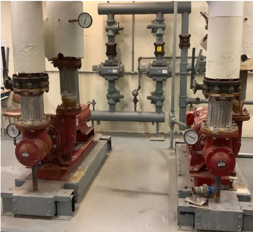
Dual Temp Pumps & VFDs
