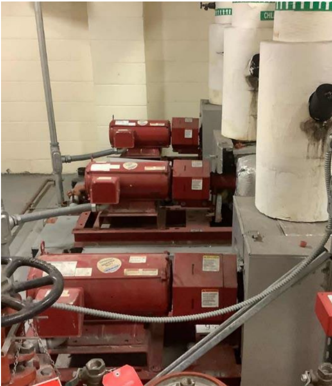
Chilled Water Pumps & VFD
