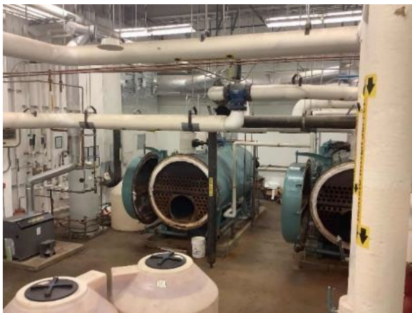
Non-condensing boilers
