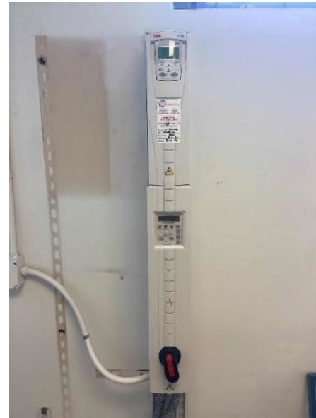
Chilled water pump VFD
