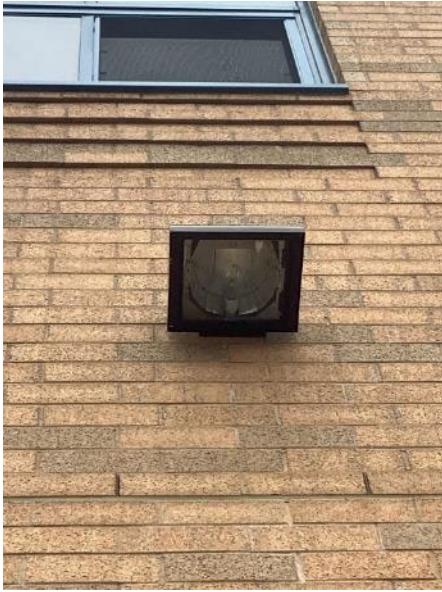
Exterior metal halide fixture
