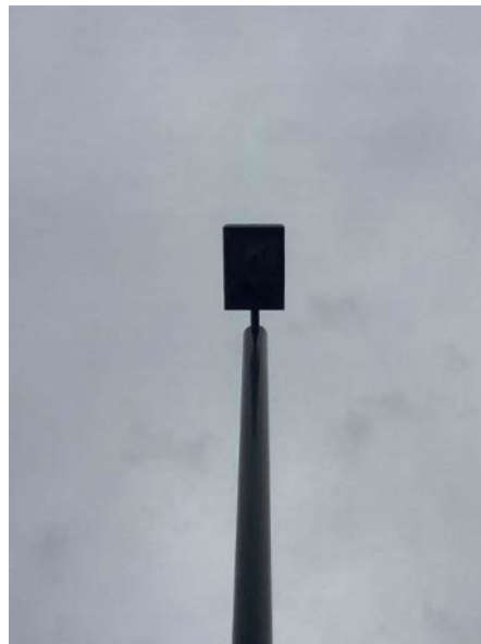
250 W High-pressure sodium pole fixture
