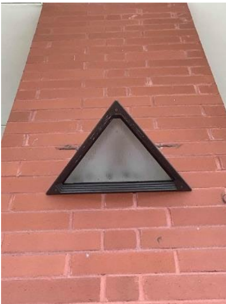
Exterior 26W CFL fixtures
