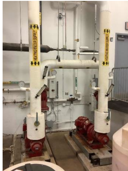
Heating hot water pumps
