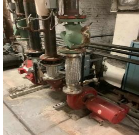
Heating hot water pumps
