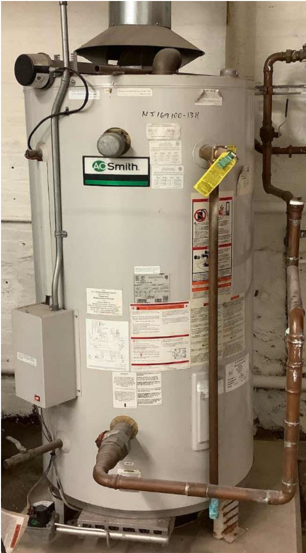
Gas-fired Storage Tank Water Heater & Circulation Pumps
