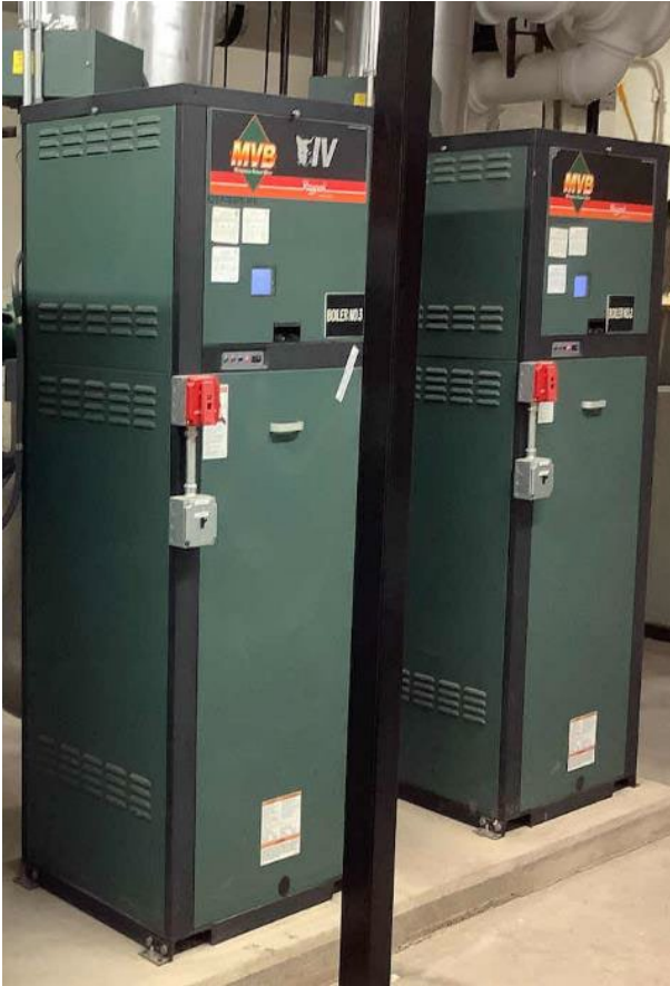
Hot Water Boilers & Hot Water Pumps
