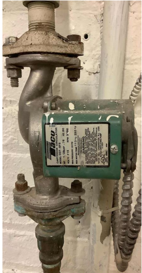
Gas-fired Storage Tank Water Heater & Circulation Pumps
