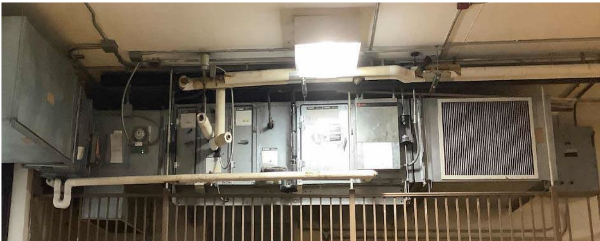
Air Handling Unit AHU-2
