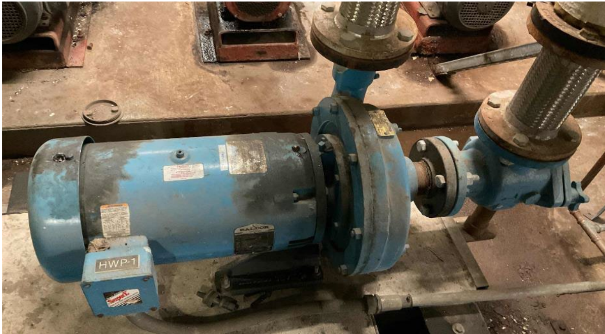
Heating Hot Water Pump
