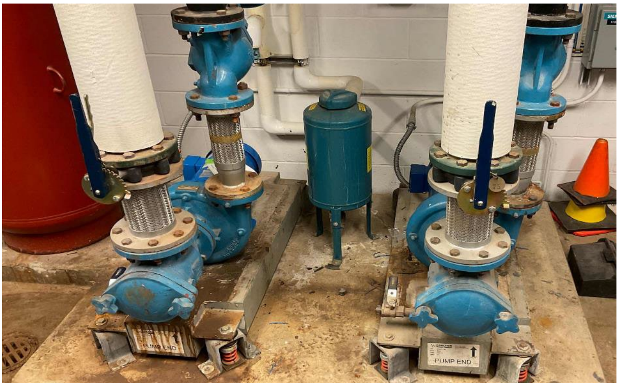
Heating Hot Water Pumps
