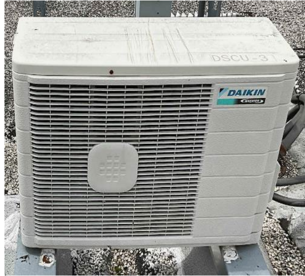
Split AC System & Mini-split HP Unit
