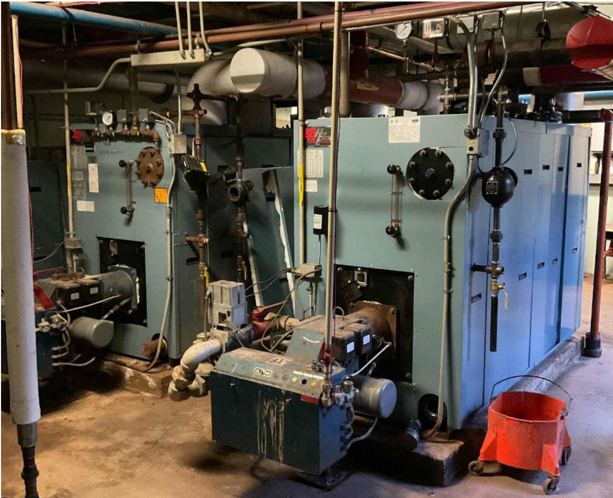
Hot Water & Steam Boilers
