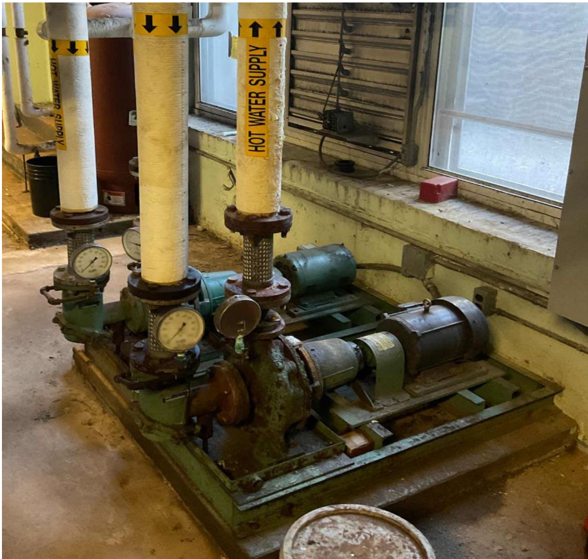
Heating Hot Water Pumps
