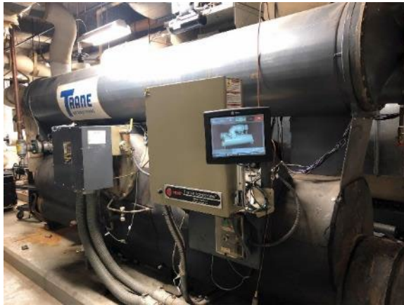
Water-Cooled Centrifugal Chiller
