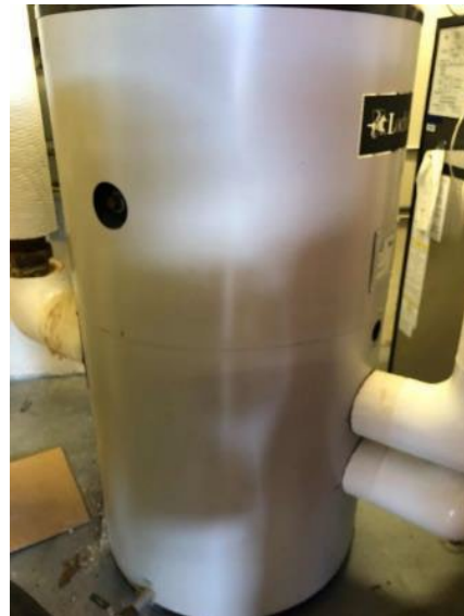
Gas-Fired Indirect System
