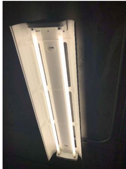
Fluorescent Linear T8 Fixture
