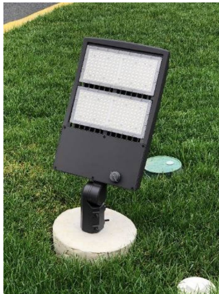
Ground Mounted LED Flood Light
