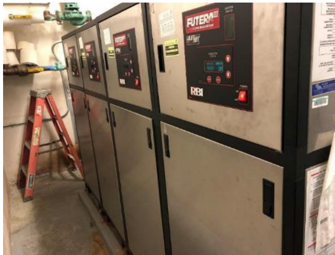
Hydronic Boiler Plant
