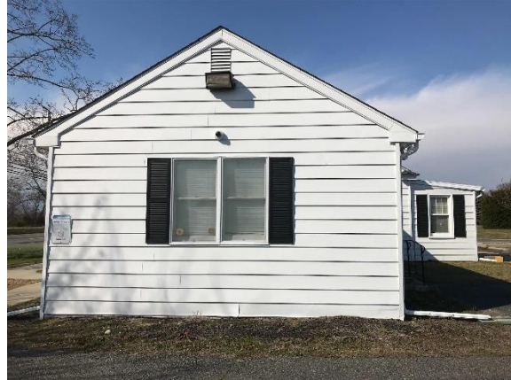
Side of Building
