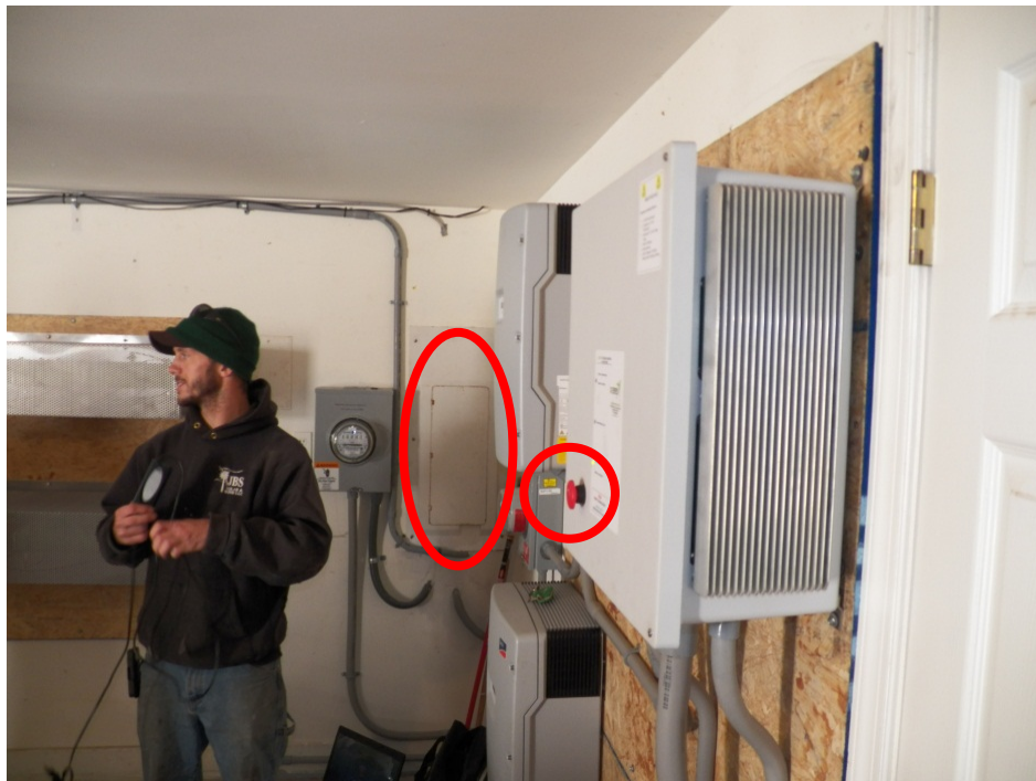
Figure 2. Turbine control box with the emergency stop button in the foreground
