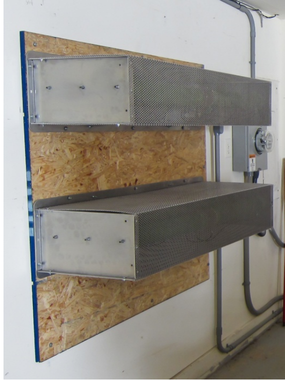
Figure 10. Mounting of diversion loads (Photo by Lee Jay Fingersh, NREL)
