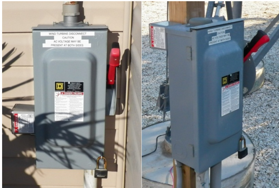
Figure 3. External turbine disconnect switches
