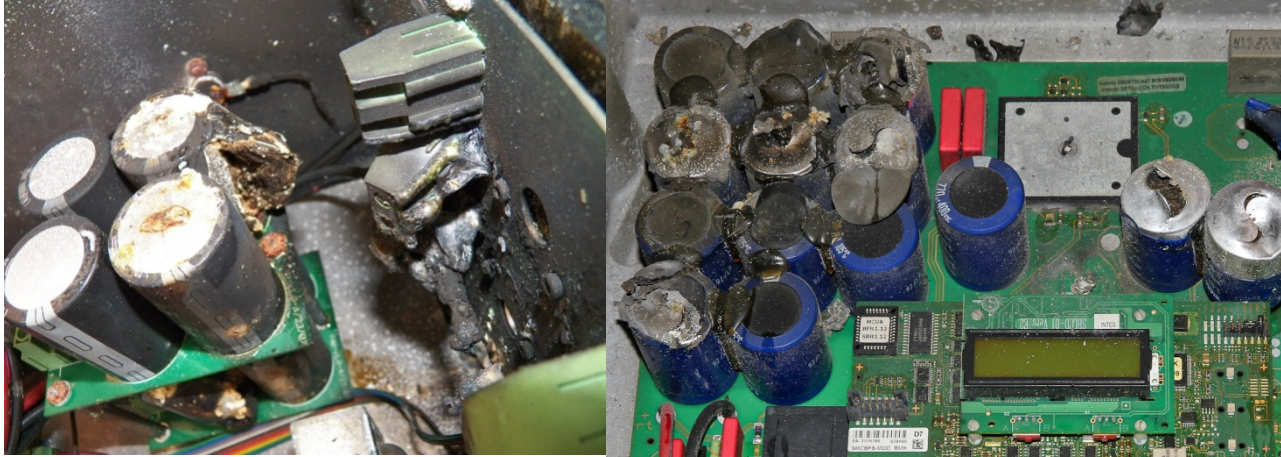
Figure 13. Capacitor failure in the turbine controller (left) and inverters (right) (Left photo by Rob Wills, Intergrid, LLC, right photo by Lee Jay Fingersh, NREL)
