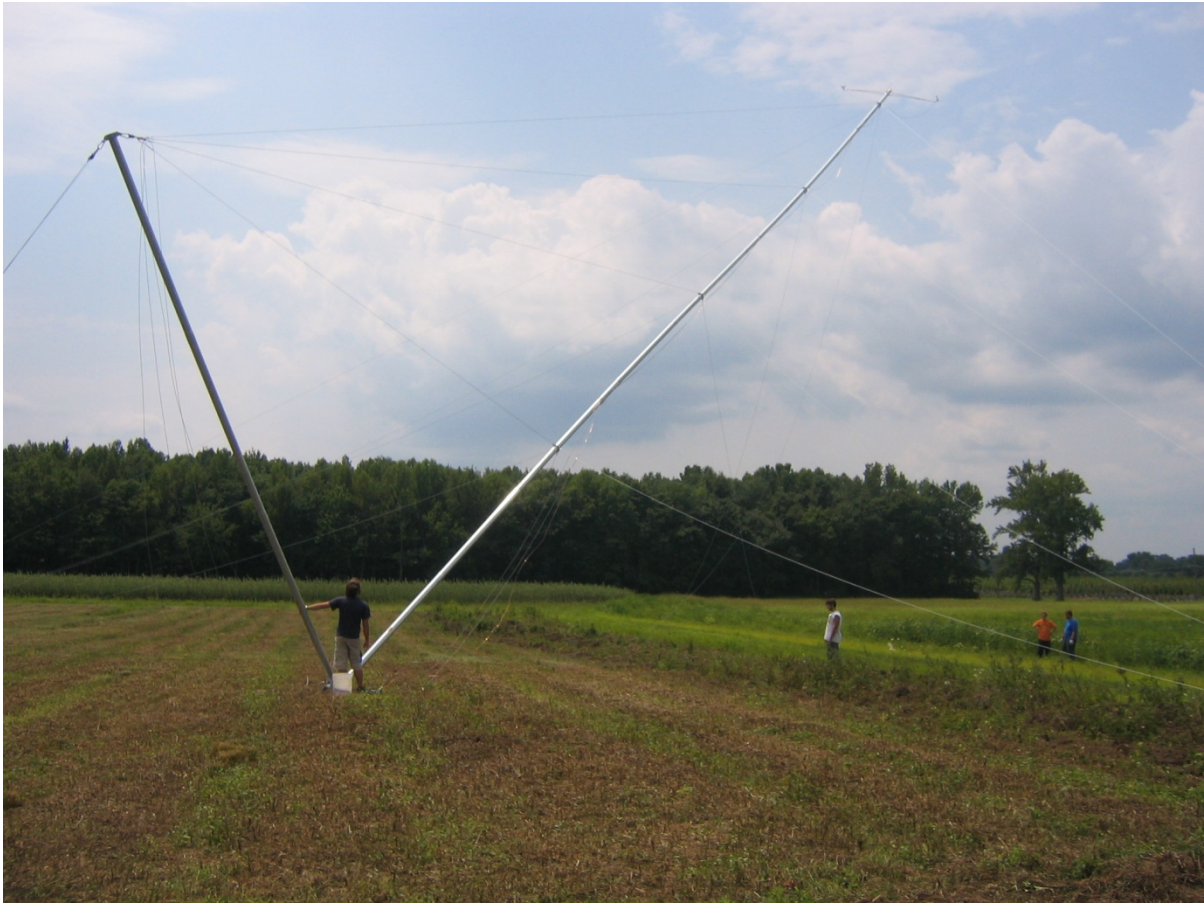
Figure 3: Tower Installation at LeBak Farms
