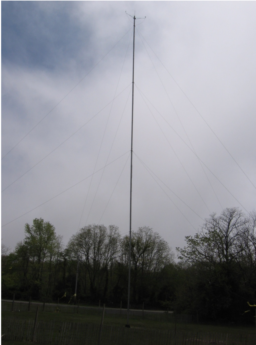
Figure 9: Tower Installation at Ocean Gate
