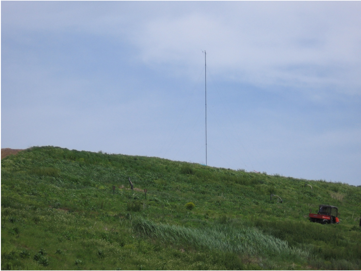
Figure 6: Tower Installation at SCUA
