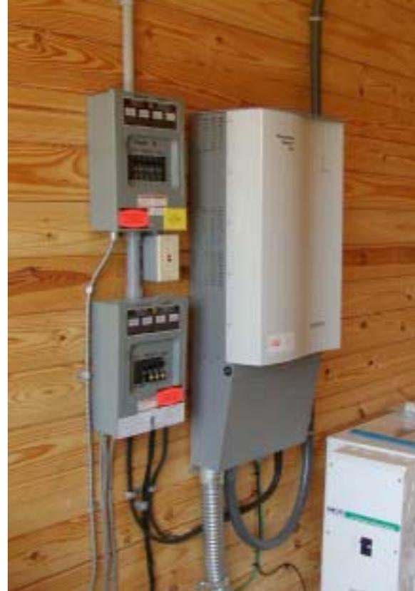
*The inverter, batteries and control equipment for the solar electric system are located inside a utility room in the barn.*
