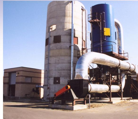
*The Rex Lumber facility houses 6 wood-drying kilns that run 24 hours a day all year. By replacing a natural gas system with a wood-waste boiler to heat the kilns, the company eliminated an average annual gas bill of \$100,000. The silo in the center stores the wood waste.*
