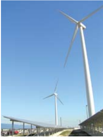
ACUA's energy initiatives included five 1.6 megawatt GE turbines installed in Atlantic City.
